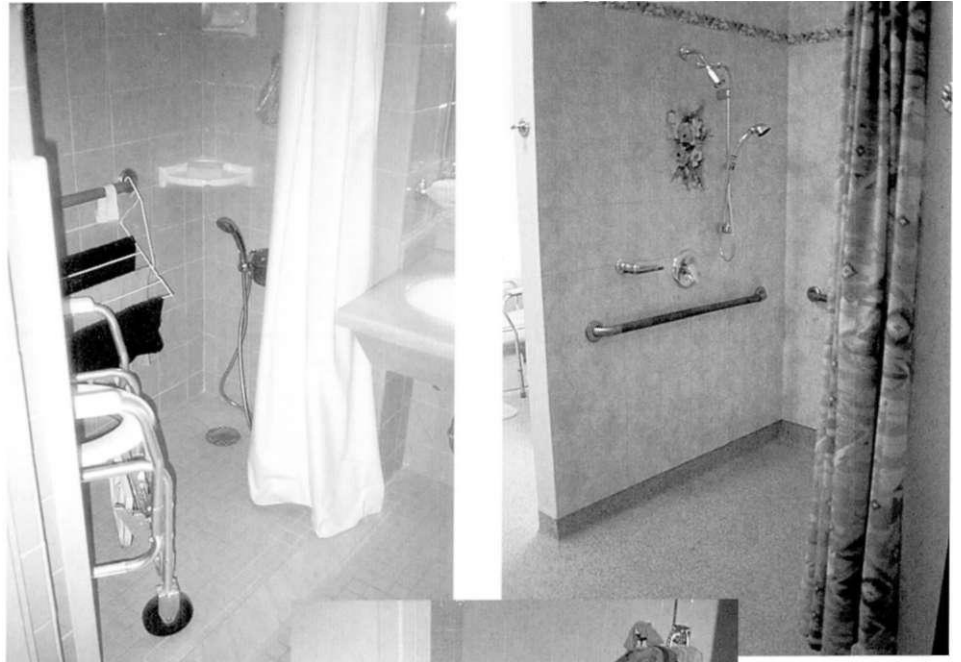
Shower floors slope down toward drain (top); mini-ramp goes up and down into shower (bottom).
