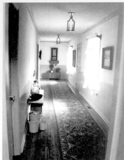
Wainscoting protects walls from damage, while wide hallway makes wheelchair travel easier.
