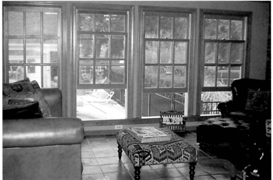
Outdoor space can be easily viewed from a wheelchair with these low windows. However, double-hung windows are difficult to open and close from a seated position.
