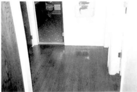
Turning space outside bathroom door.
