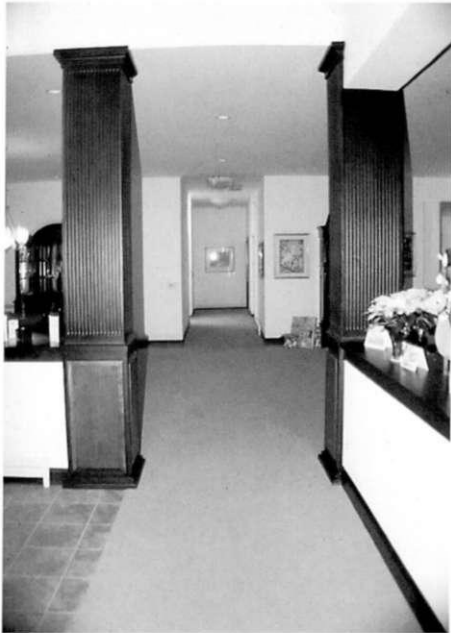
Wide hallway increases wheelchair access.
