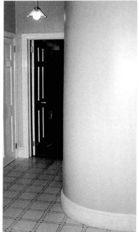
Curved wall (above) and angled wall (right) can ease wheelchair turns.
