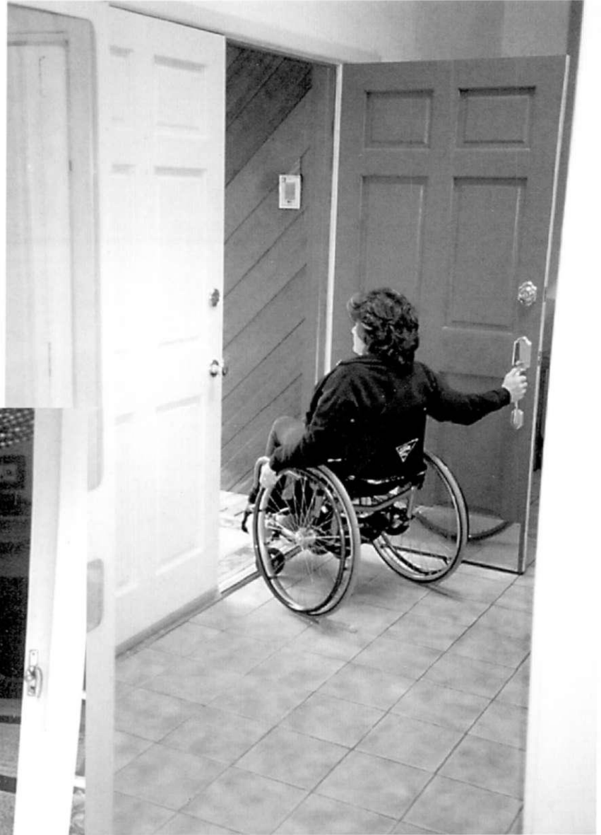
Doorway with minimal threshold.
