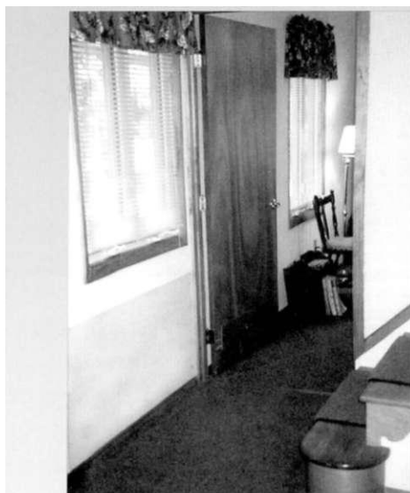
Plexiglass panel beneath window protects the wall.
