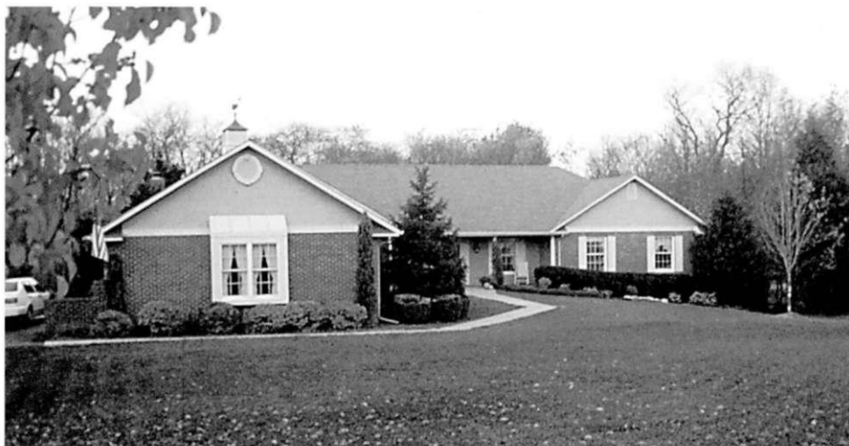
Accessible walkway extends around the exterior of the house.
