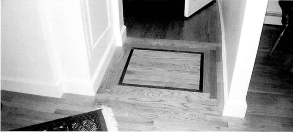
Attractive hardwood ramp eliminates step to a "sunken" room.
