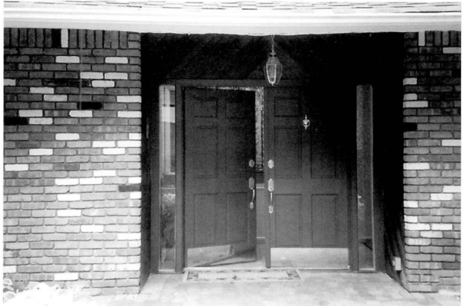
Double doors create a very accessible entry.
