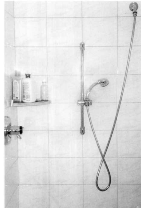
Adjustable height shower head slides along vertical bracket.
