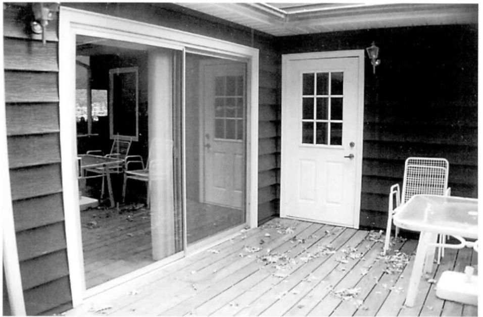
Sliding doors create a wide entry.
