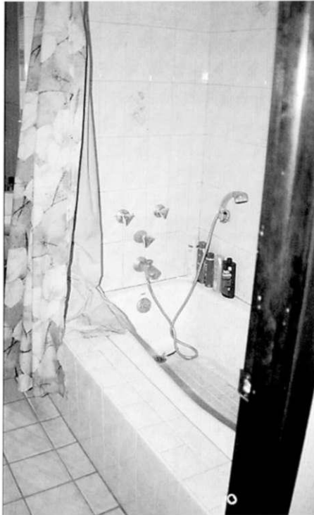
Wide ledge along side of tub helps with transfers and provides place for a parent to sit.
