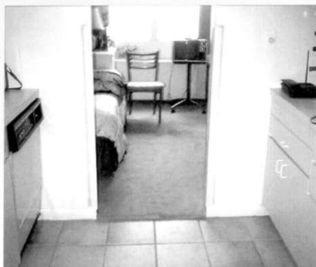
Plastic corner guards cover a door frame.
