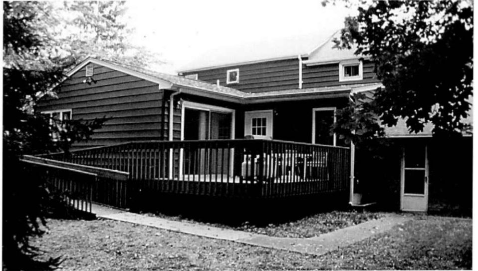
Rear deck and ramp provide a second accessible entry and exit.
