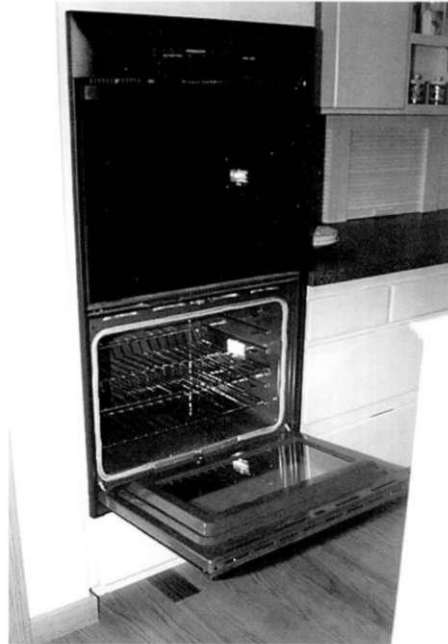
Oven at wheelchair height, but bottom-hinged door blocks access.
