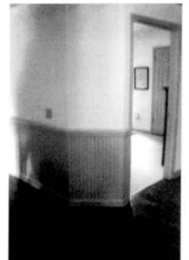
Curved wall (above) and angled wall (right) can ease wheelchair turns.
