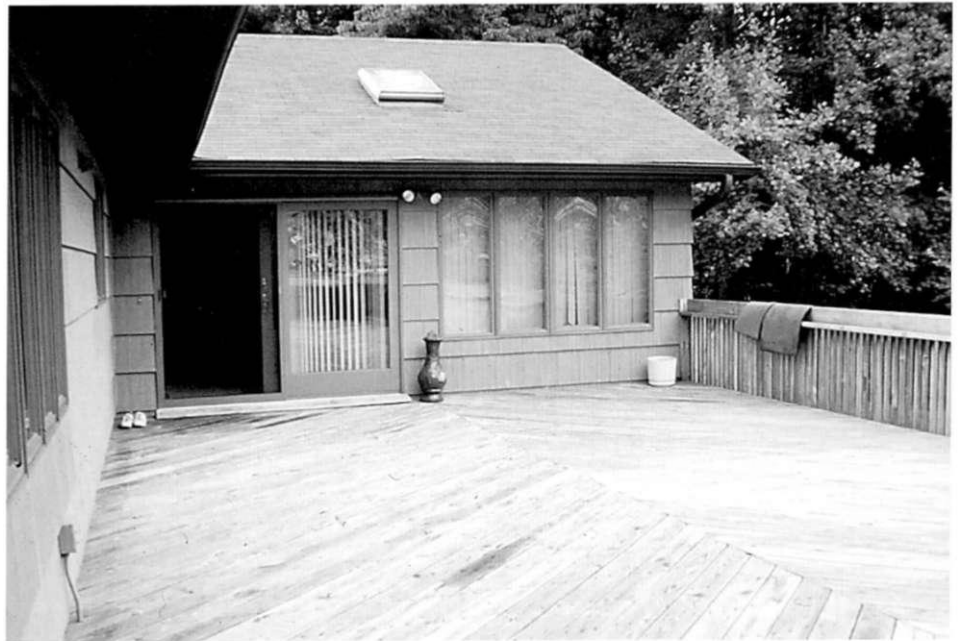
Wide sliding door opens onto large wooden deck.
