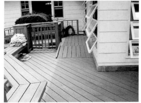
A ramp placed too close to windows that open outward can be dangerous.
