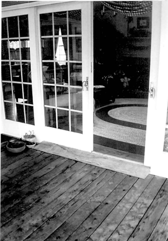
Mini-ramp for rolling chair over doorsill.
