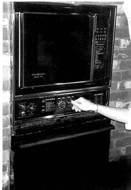
A combination with low oven and a microwave above and controls in between makes an accessible cooking unit.
