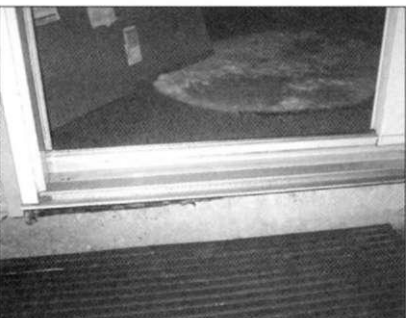
High thresholds at doorways are hard to negotiate.
