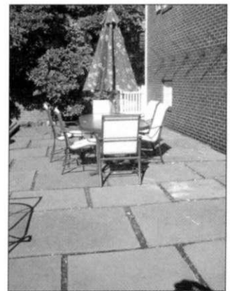
Be careful with spaces between pavers. They can be tripping hazards.
