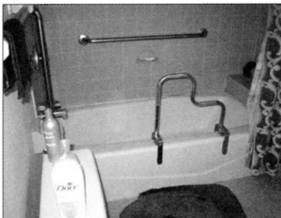
A grab bar that takes up too much room can make it hard to climb in and out of the tub.
