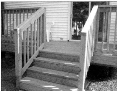
Plank railings are hard and uncomfortable to grasp.
