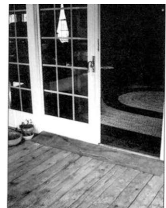
A threshold ramp removes a tripping hazard and makes the door more accessible for people in wheelchairs.
