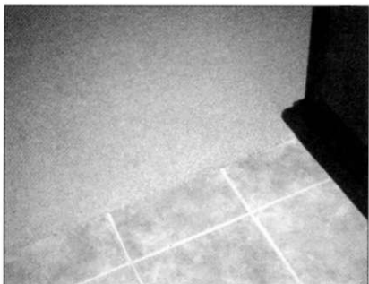
Smooth transitions between flooring surfaces eliminate a tripping hazard.
